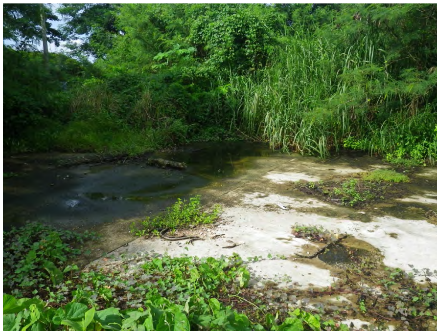
FIGURE 7-18. CONCRETE PAD, FEATURE 9.
