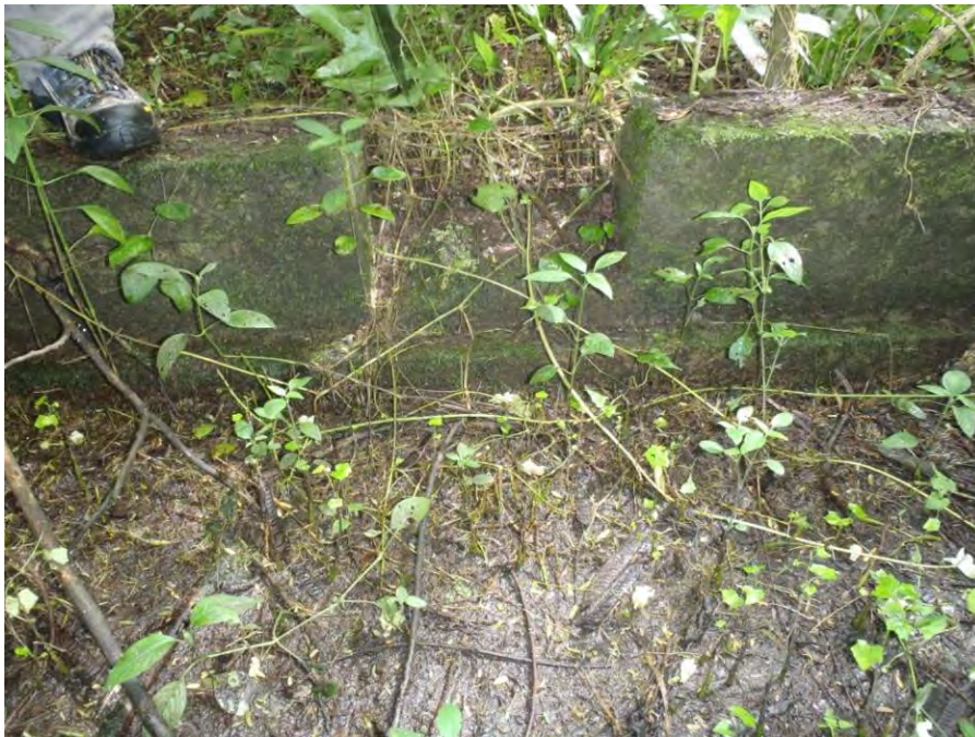
FIGURE 7-7. FEATURE 3 DETAIL OF CONCRETE PIT EAST WALL.
