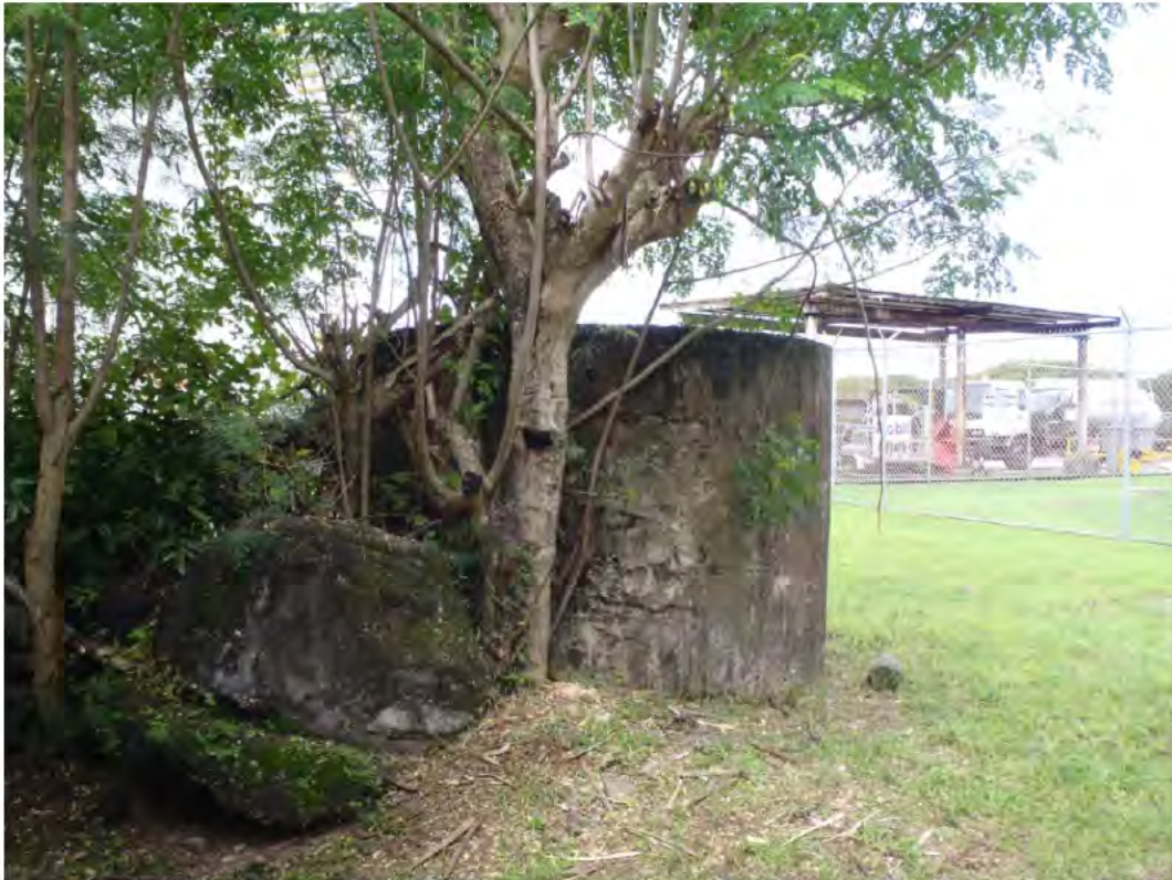
FIGURE 7-5. VIEW SOUTH OF WATER RETENTION STRUCTURE (FEATURE 1).
