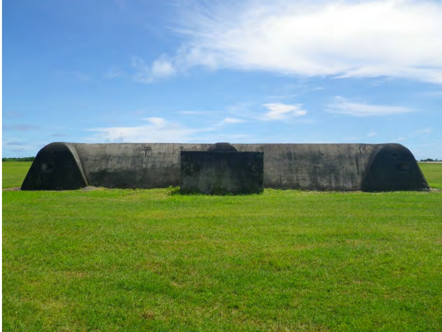
FIGURE 7-24. VIEW SOUTHEAST OF BUNKER AB2.
